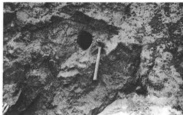
Photograph 2 - Detail of a tubular cavity.
