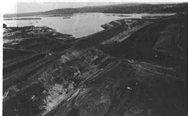
Photograph 1-Partial view of Tucuruí Dam's construction
