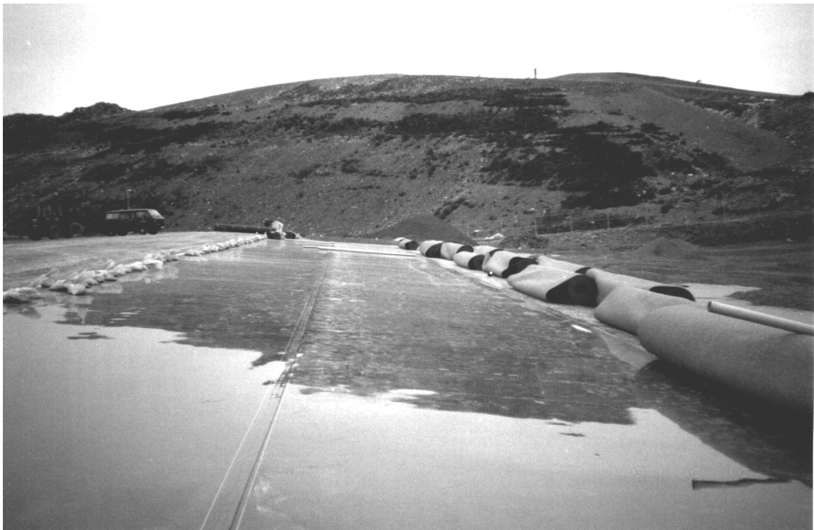
Figure 6. Example of a flat geomembrane on a landfill bottom.
