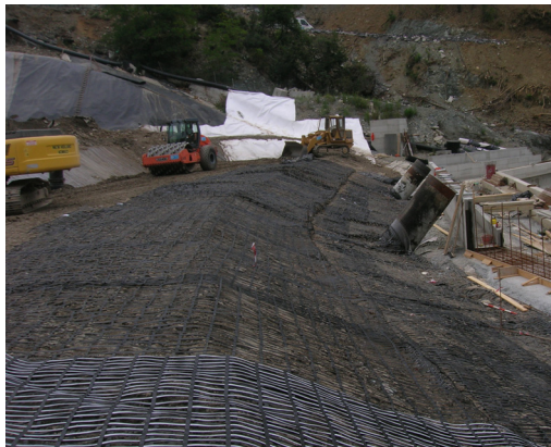
Figure 1 Construction stage of the embankment.
