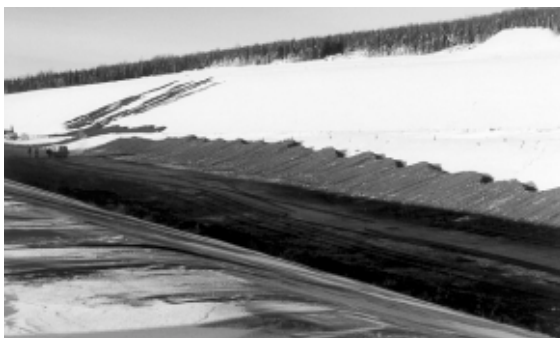
Figure 1. Solution trough at low end of leach pad.
