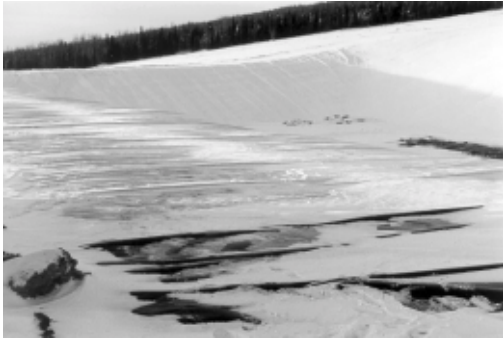
Figure 2. East end of Cell. Black uppermost in foreground. Beige on top in background. Liner is not under tension.
