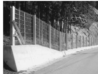
Photograph 2. An existing stone guard fence
