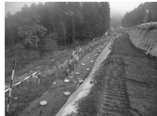
Photograph 2. Install the pile
