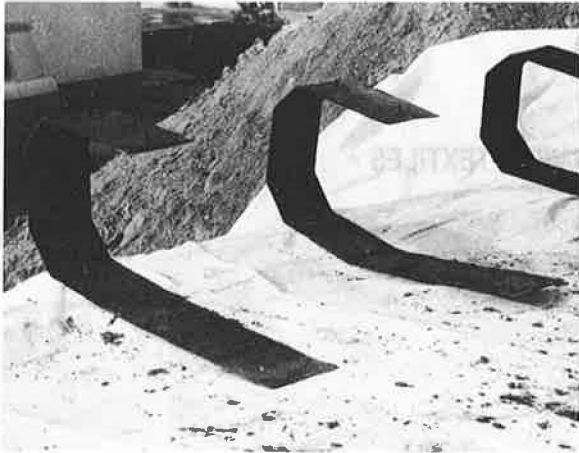
Fig. 2 Edged rigid metal lengths used as stabilizers which remain in the structure
