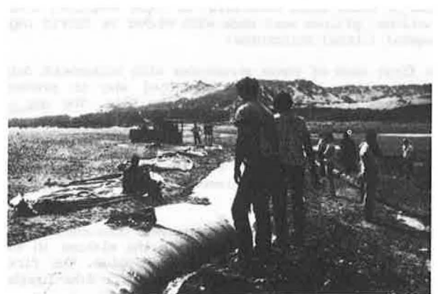
photo 3 : Filled fabric tube of SLACK bay dike
