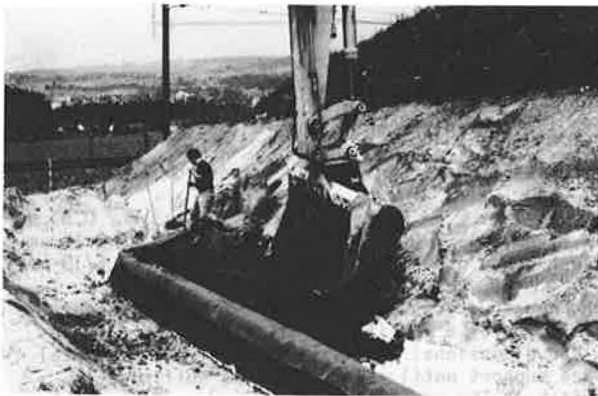
Photo no. 2: Placing the initial layer
