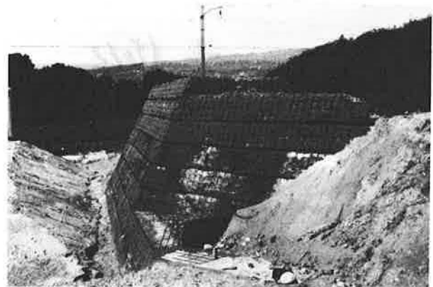
Photo no. 5: Test slope immediately after construction
