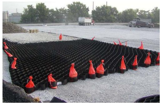
Figure 1. Geocell reinforcement road and subgrade applications
