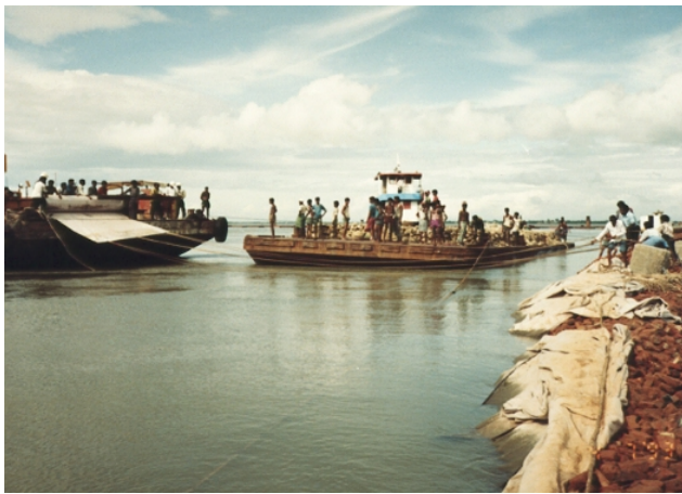
Figure 13. Dhaka : installation of the ballasted filtration geotextile
