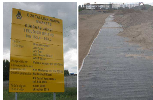
Figure 1. Building site sign and geogrid installation
