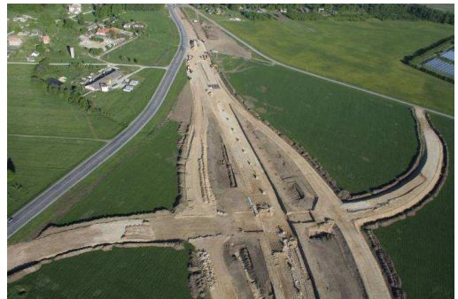
Figure 6. Aerial view of the building site.
