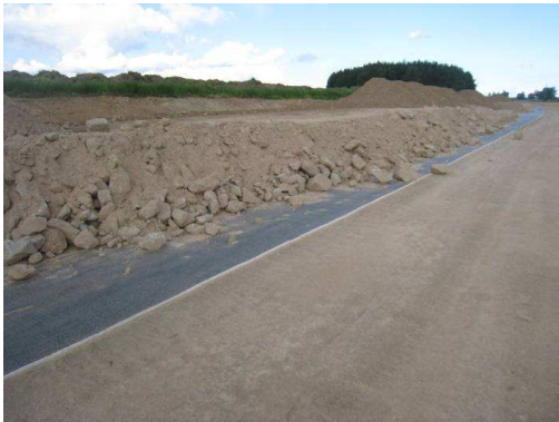
Figure 8. Geogrid starting to be covered.
