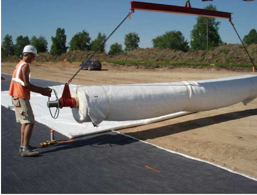
Figure 7. Installation of the geogrid.
