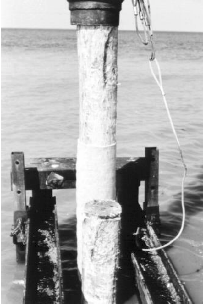
Figure 6: Installation of geotextile-covered groyne piles by rammer off Kuehlungsborn (Mecklenburg-Vorpommern)
