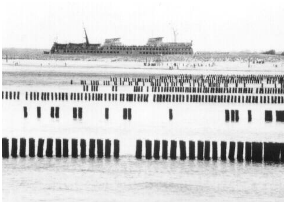
Figure 1: Loss of piles in the groyne field off Rostock (Sordyl et al. 1998)
