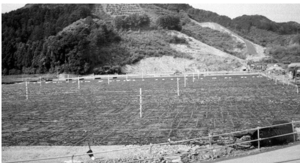
Photograph 2. Installed situation (approx. 9000m 2 )
