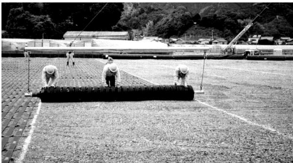
Photograph 1. Installation work of geosynthetic
