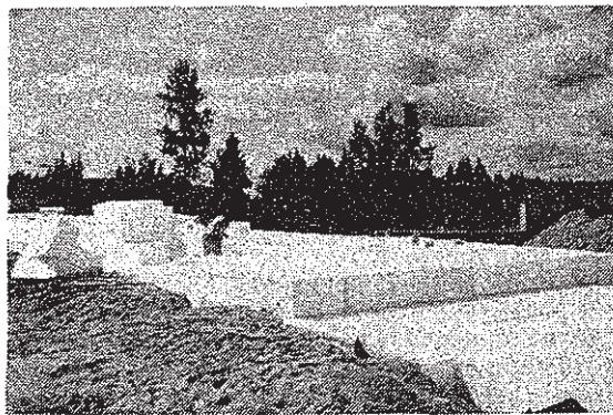
Fig 1. EPS blocks in roadfill.
