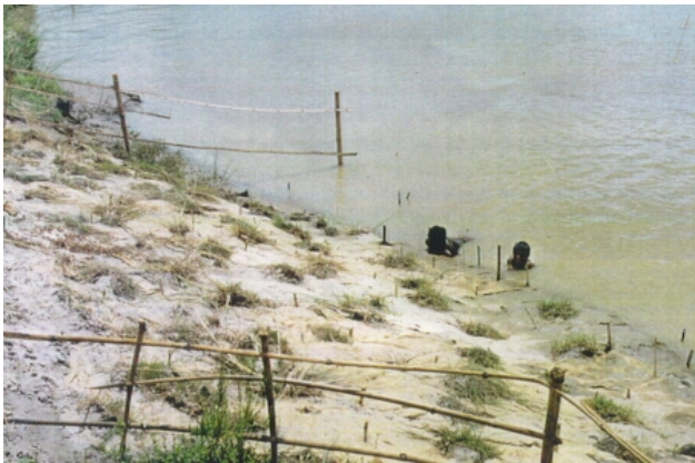
Photo 2. Geo-Jute nonwoven to control erosion (Charkrishnabati)
