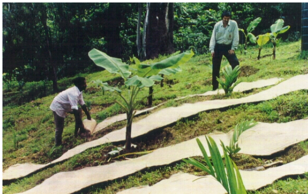
Photo 3. Application of geomat in progress (Andaman)
