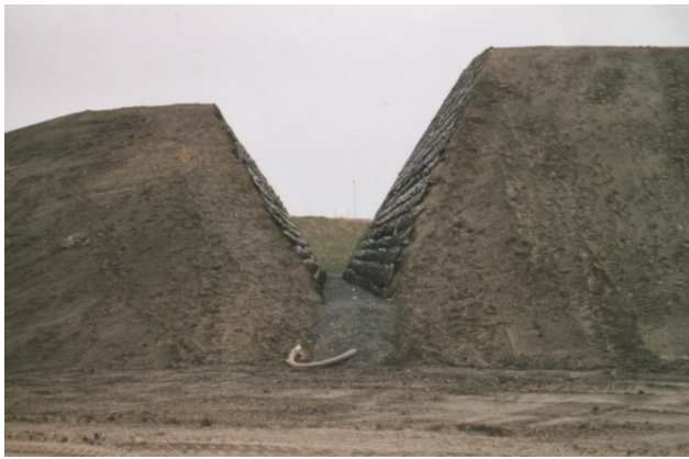
Photo 3: Cleft after finishing construction
