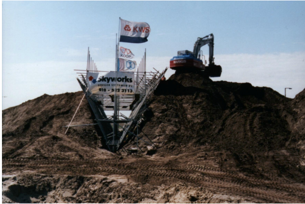
Photo 2: Scaffolding during construction
