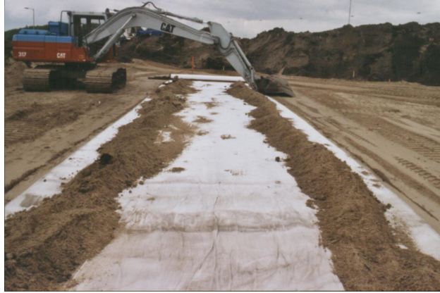
Photo 1: Placing high strength basal reinforcement
