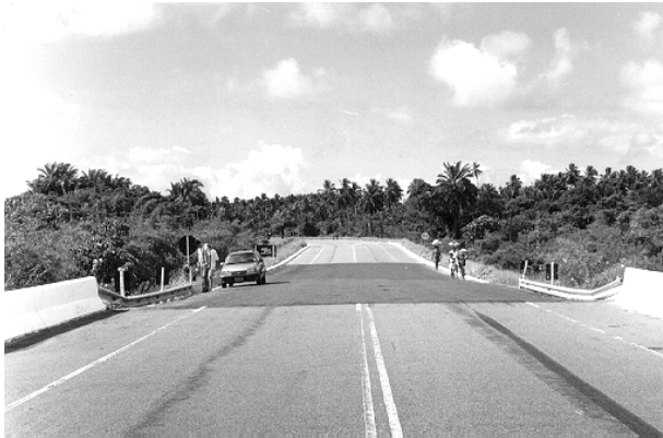
Figure 12. Repairs in the pavement of Case History 4.
