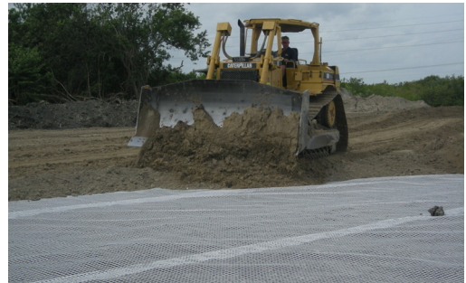
Figure 13 Installation of geocomposite reinforced piling platform
