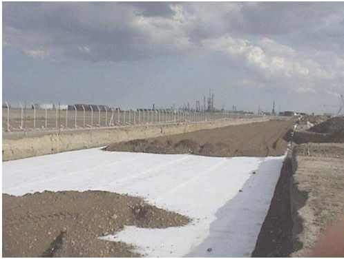
Figure 12 Installation of composite base course reinforcement
