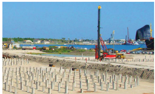
Figure 14 Piling works in the area of planned fuel tanks
