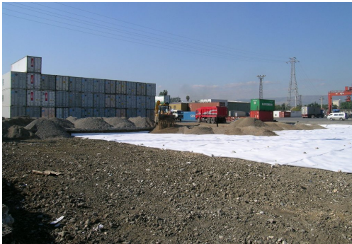
Figure 10. Installation of composite base course reinforcement
