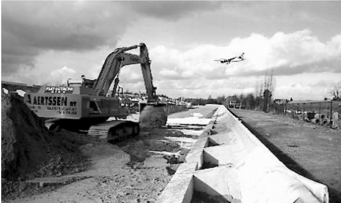
Figure 6. Reinforcing geotextile is hung out over the face of the slope whilst sand is built up within and behind the element.
