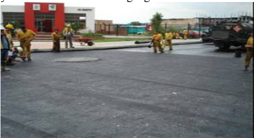
Picture 3. Roadwork after fiberglass application
