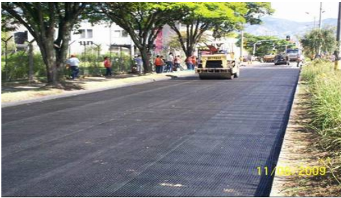
Picture 2. Roadwork after fiberglass application
