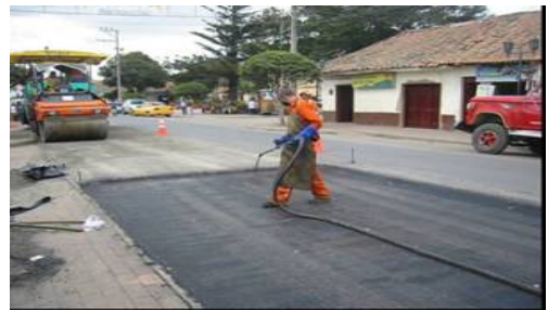
Picture 1. Roadwork after fiberglass application.
