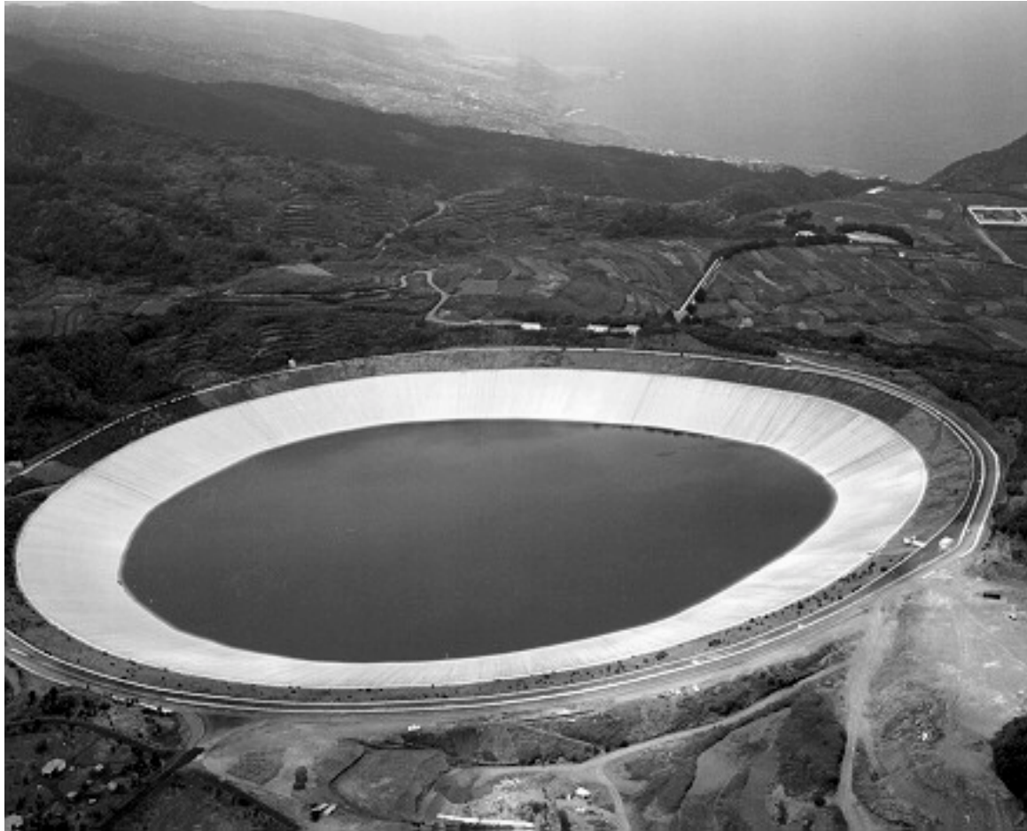
Figure 8: Barlovento Reservoir; Canaries Island PVC geomembrane 1.5 mm, 1991
