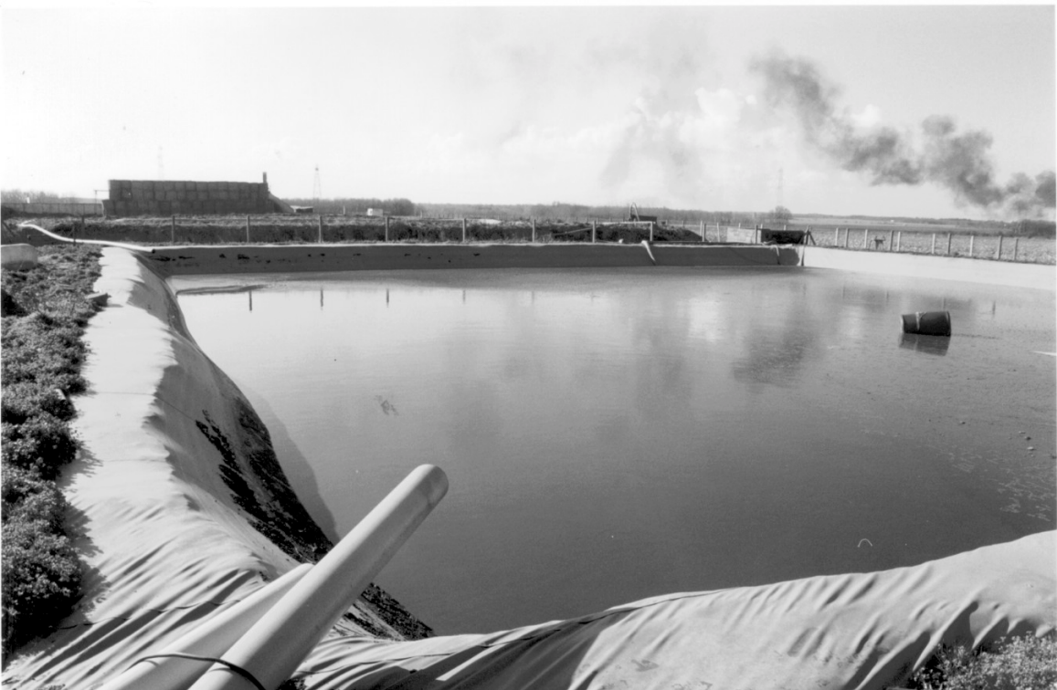
Figure 3: Mar cay Pond (1981/1982); irregularities of supporting layer
