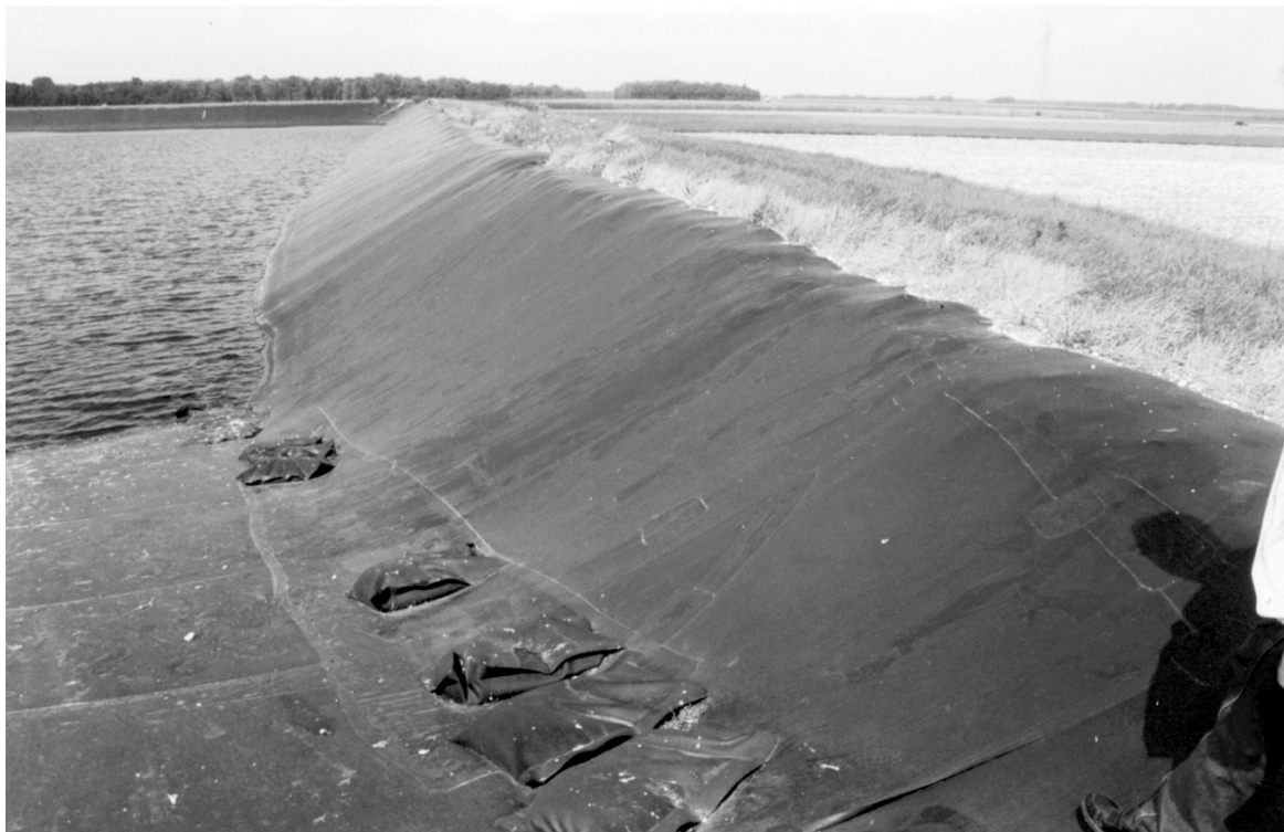
Figure 6: Préfontaines, detail of access ramp; note horizontal welding (right)
