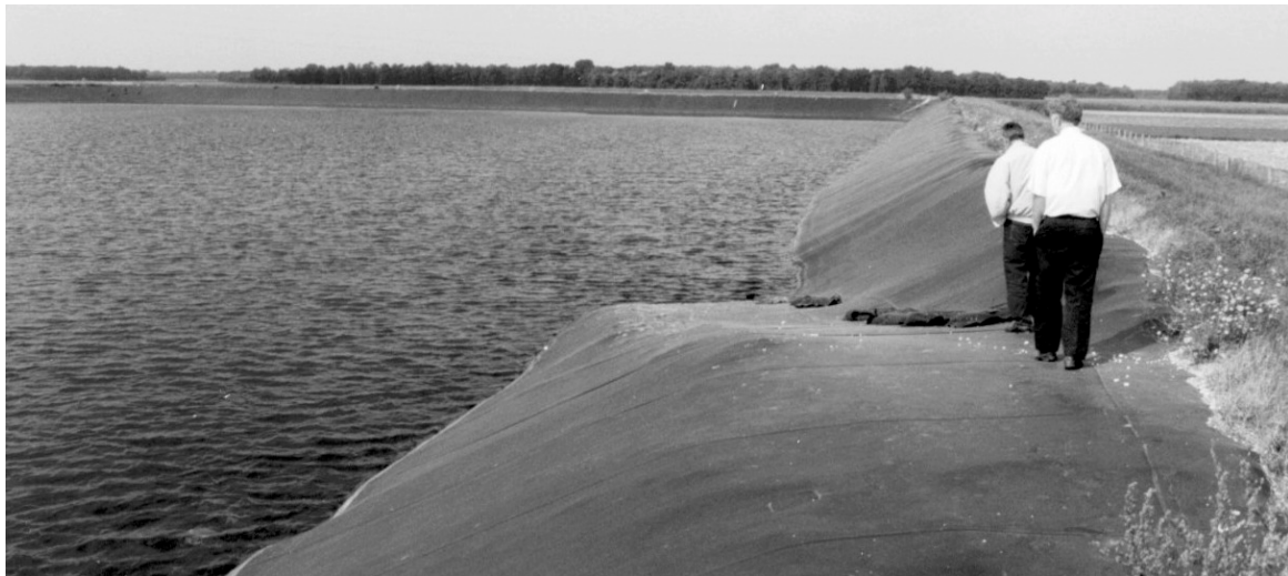
Figure 4 Préfontaine PVC 1mm thick 40000 m 2 1982; view after 18 years
