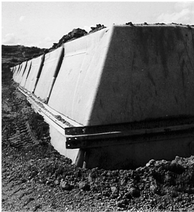
Figure 4: External bund segment with guard board; filled with cohesive soil
