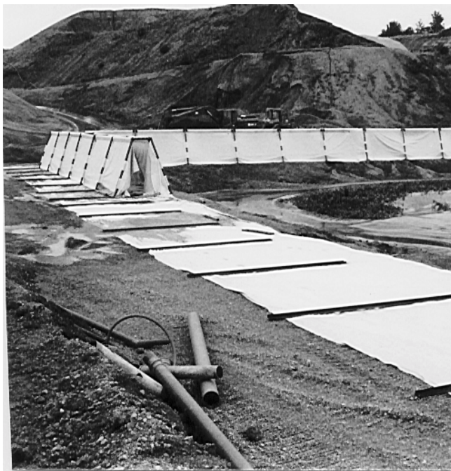
Figure 3: Bund elements during construction
