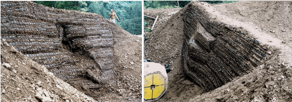
Fig. 9: Views of front and back deformations after the first impact in the 4354 kJ test.
