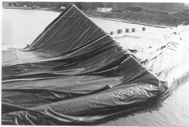
Figure 2 Sinking the membrane from a pontoon
