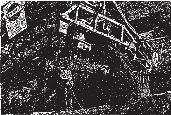
Mixing of soil and yarn by special machines.
