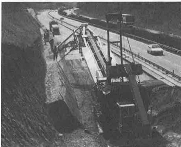
Figure 11 - View showing a close-up of the retaining structure being constructed
