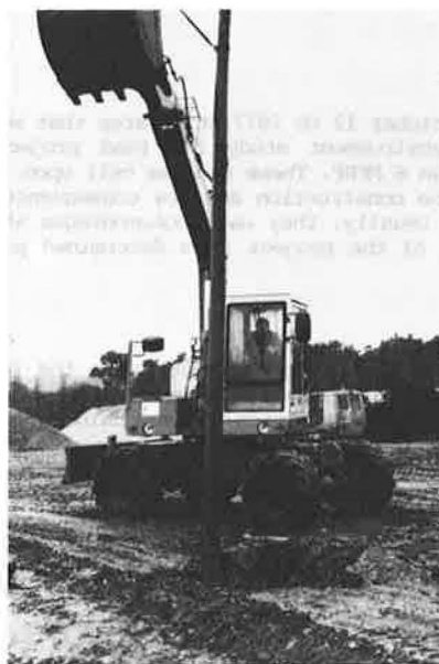
photo 2 : Installation of the mats use of hydraulic shovel
