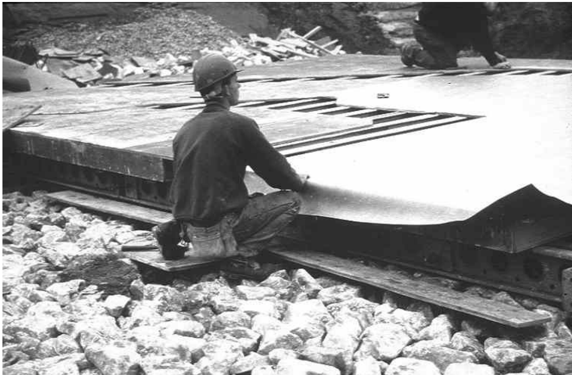
Figure 4. Fixing the textile to the wooden formwork. Stapling edges.
