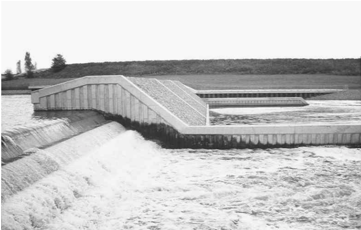
Figure 2. Photograph of weir with central siphon section at normal flow level.
