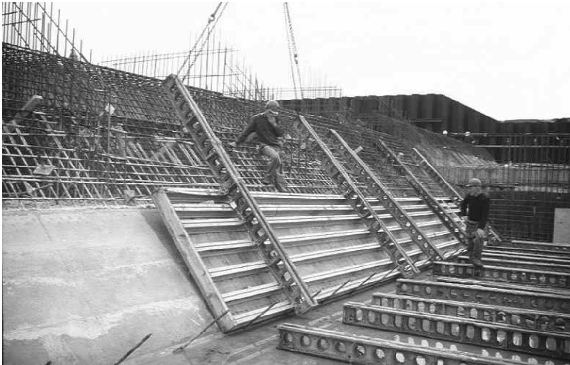
Figure 5. Sloping formwork being removed from a moulding.
