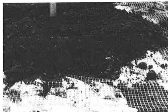
Photo. 2 Surface of P section reinforced with polymer grid
