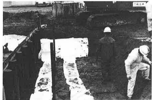
Photo. 1 Placing non-woven filter fabric for horizontal drainage
