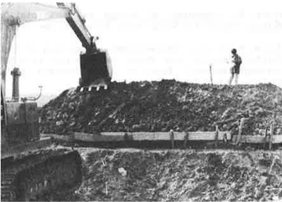
Photo. 4 Completion of pre-loading soil of 2 m height for consolidation of sludges
