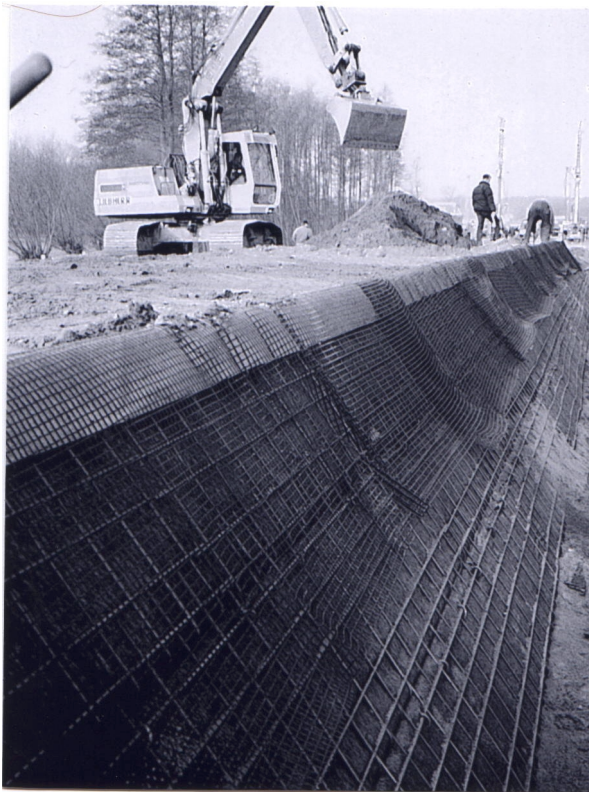
Figure 5. State of construction work on over-steep slopes
