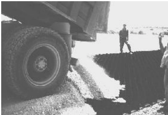
Figure 7: Filling granular material.
