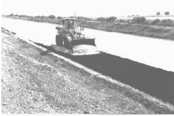
Figure 8: Filling granular material.
