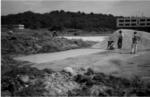
Figure 1. On site work phases
