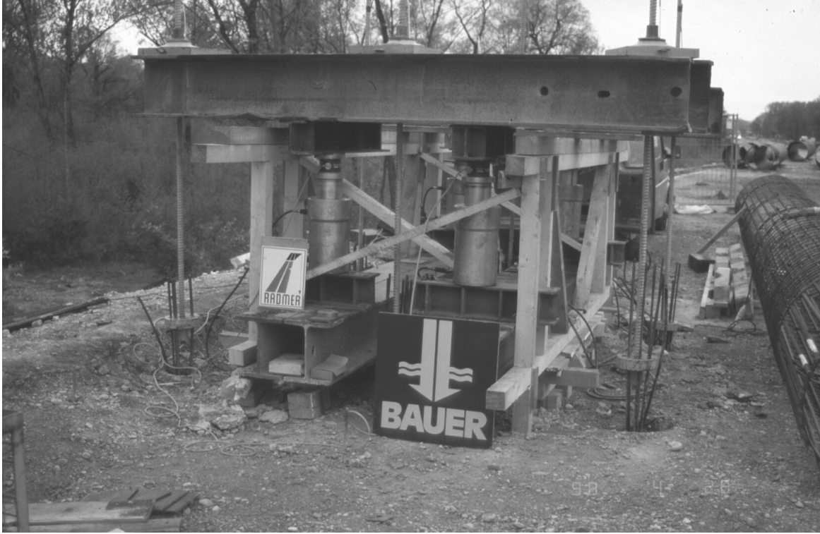
Figure 8: Ground anchors as abutment for test loading of the reinforced slope
