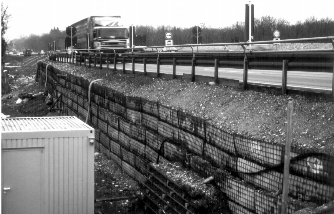
Figure 6: Temporary reinforced slope under heavy motorway traffic
