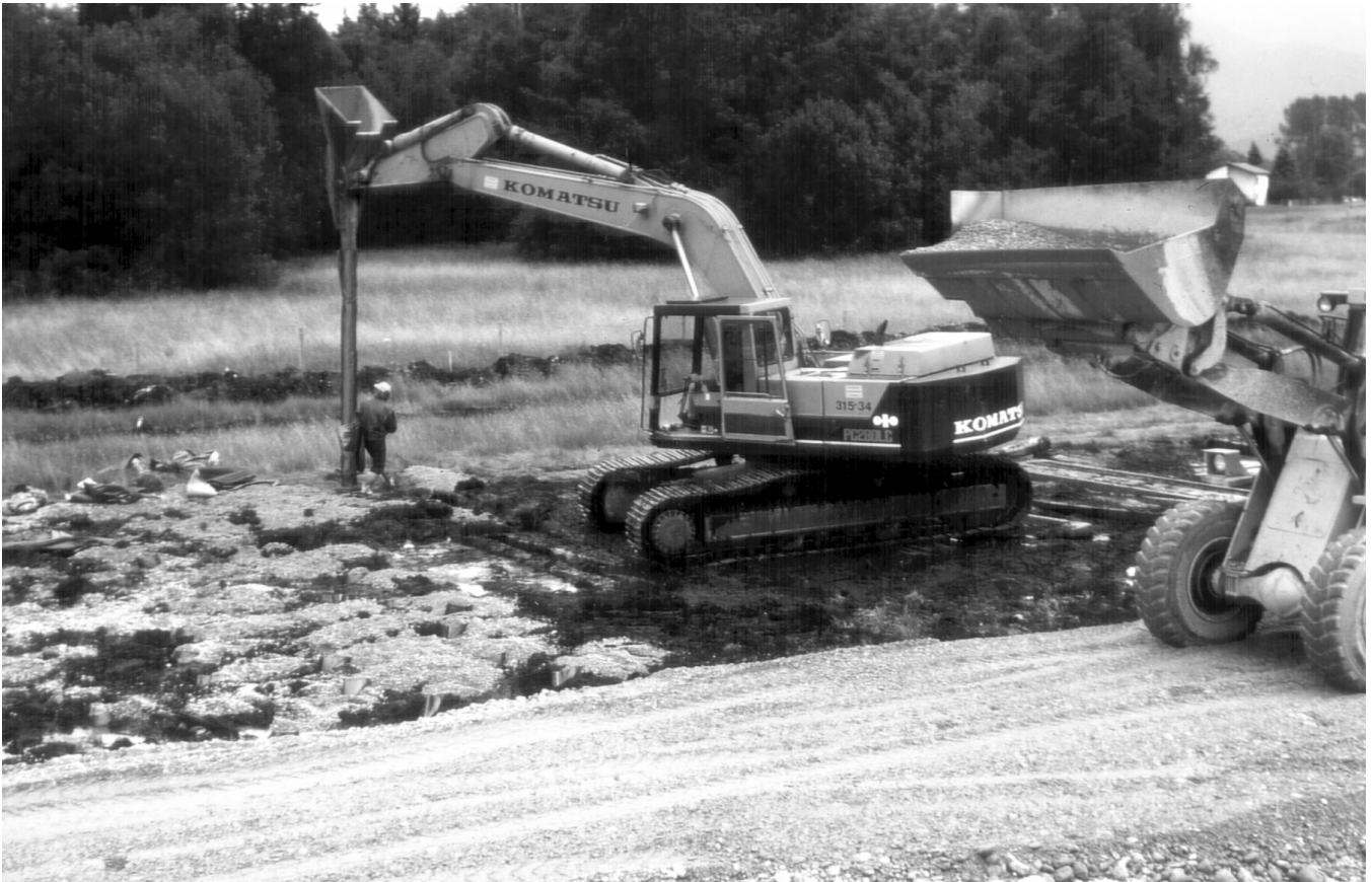
Figure 1: Installation of geotextile coated gravel columns
