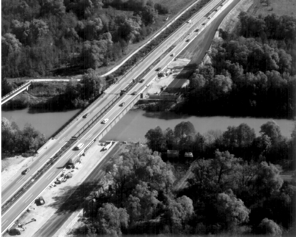
Figure 5: Location for temporary reinforced slopes at river “Tiroler Ache” within nature reserve areas
