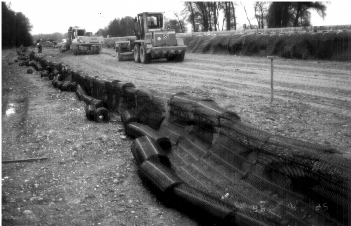
Figure 4: Installation of “gravel mattress” within former pond
