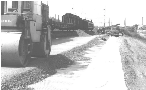
Figure 4. Geogrid and underlying GCL placed on subbase
