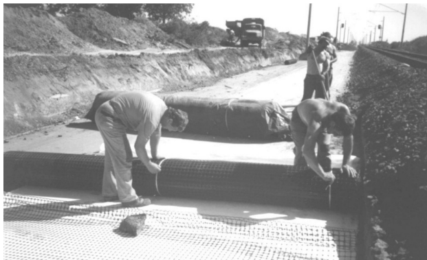
Figure 8. Placement of stiff geogrid. Line No.1
