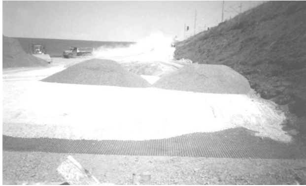
Figure 7. Widening of the embankment
