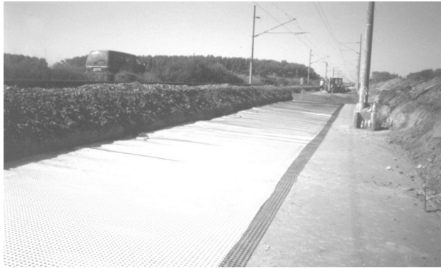
Figure 9. Site before placement of subgrade layer. Line No.1
