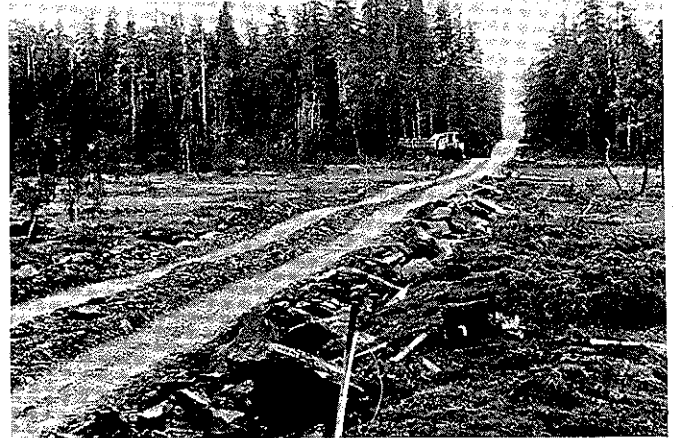
Figure 2. Immediately after construction.
