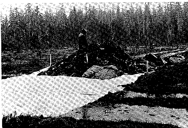
Figure 1. Road during construction.
