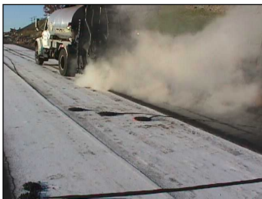
Figure 4. Applying tack coat on top of the geocomposite membrane
