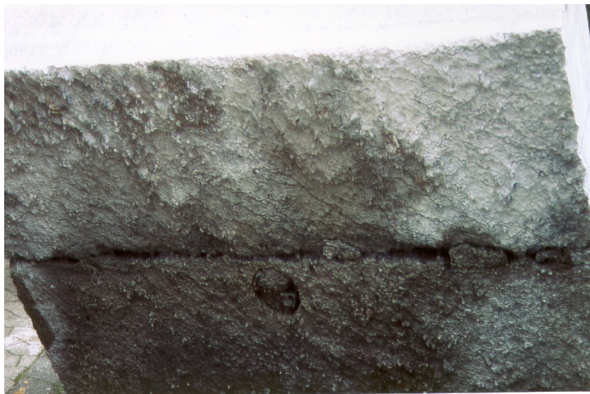
Fig. 8: View under a lifted concrete plate with partially attached THB
