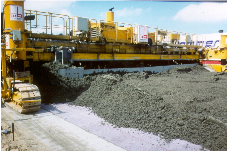
Fig. 7: Installation of the concrete surface on nonwoven fabric
