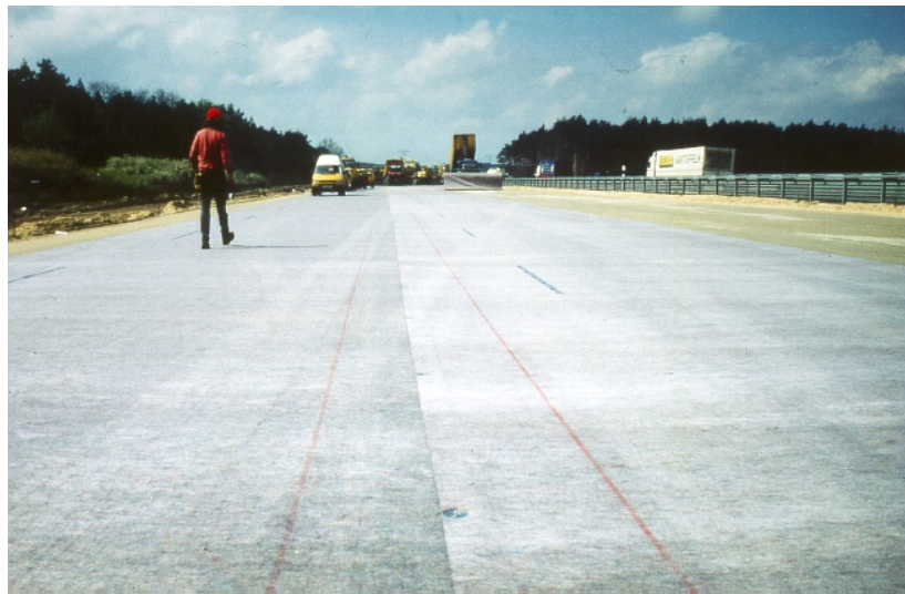
Fig. 6: Nonwoven fabric laid over the entire area
