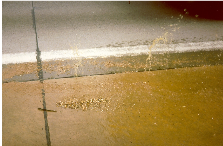
Fig. 1: Water being ejected from the longitudinal joint between roadway and hard shoulder together with fine particles and sand from the THB
