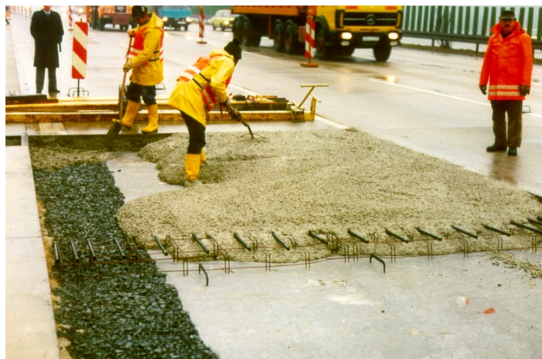
Fig. 5: Installation of the concrete on nonwoven fabric with longitudinal drainage
