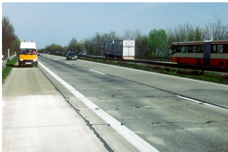
Fig. 2: Concrete surfaces on a federal motorway shortly before being renewed
