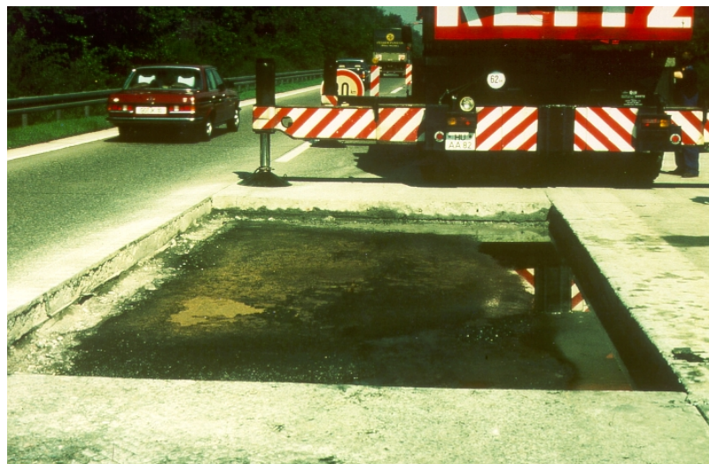
Fig. 3: Water build-up and erosion of the ATS in front of a marginal strip
