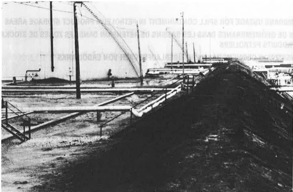
Figure 1: Conventional Berm Containment
