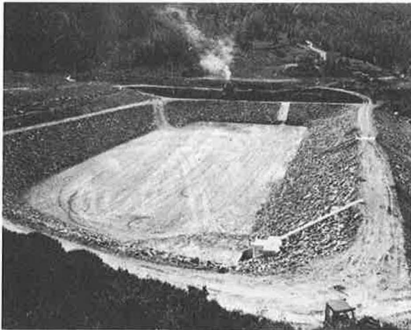
View 4 - Riberole reservoir before water filling
