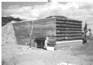
Photo 12 The completed reinforced earth, 1996
