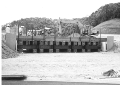
Photo2 Placement of H-section steel beams
