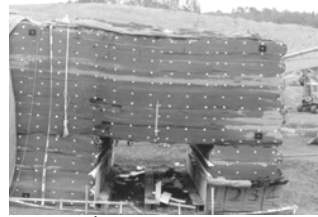
Photo 14 Completion of the soil bridge
