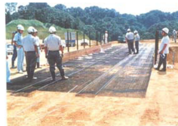
Photo 3. Placement of the geogrid
