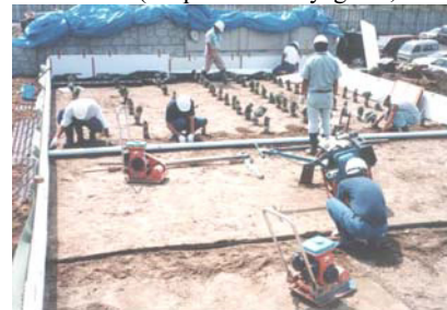
Photo 10. Construction works going on, 1996
