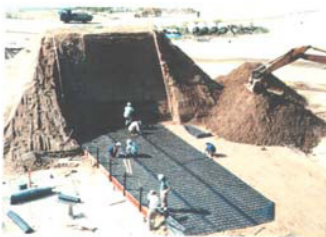
Photo 5 Start of the construction, 1993
