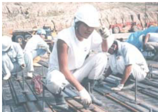
Photo 11. Pre-stressing the reinforced earth
