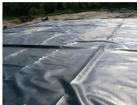
Figure 2. Interconnected wrinkles in a GM; midmorning when ambient temperature is 17°C (same location as shown in Figure 1)
