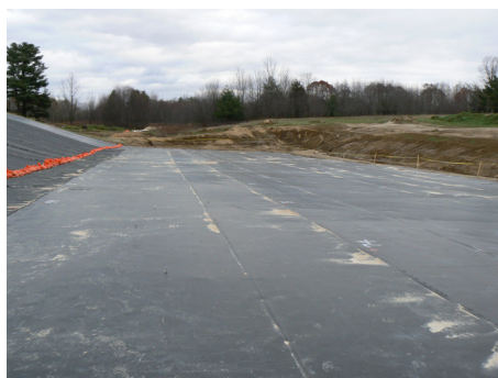
Figure 1. GM with essentially no wrinkles (in direct contact with the underlying clay liner); cloudy early November morning when ambient temperature 3°C.
