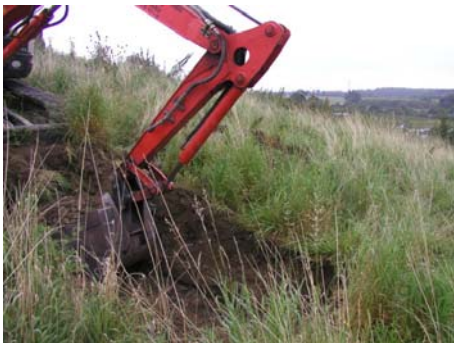
Figure 7: Excavation on landfill C
