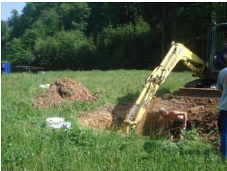
Figure 5: Excavation on landfill B
