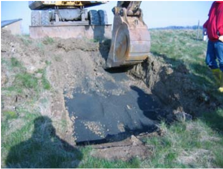
Figure 3: Excavation on landfill A
