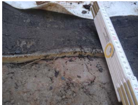
Figure 6: Cut GBR-C and subgrade in landfill B
