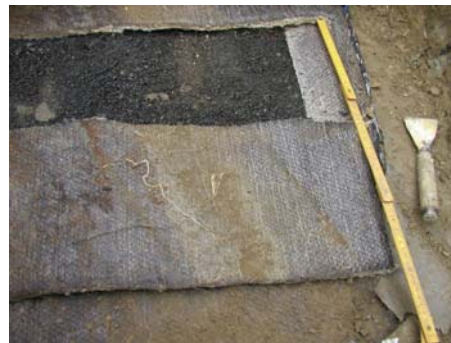
Figure 8: GBR-C with roots and subgrade in landfill C
