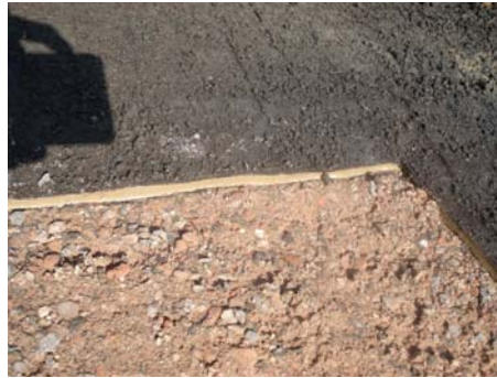
Figure 4: Cut GBR-C and subgrade in landfill A
