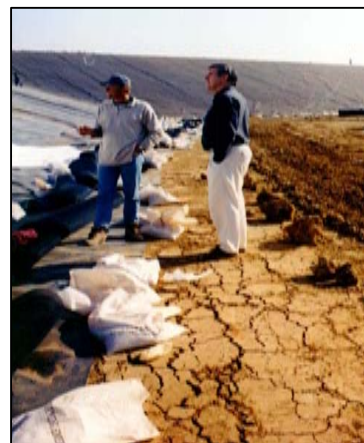
b) Insufficient surface, desiccation
