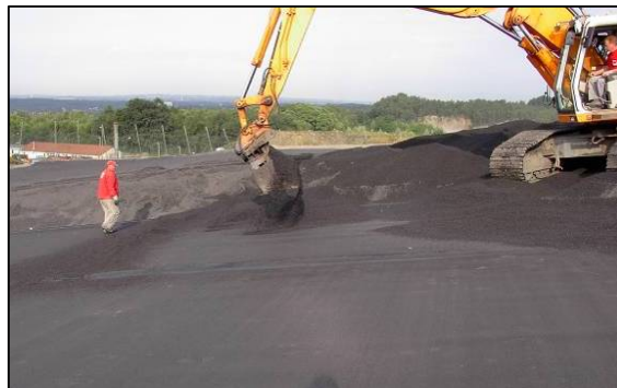
Figure 4. Installation of mineral layer with long-arm excavator from a ramp
