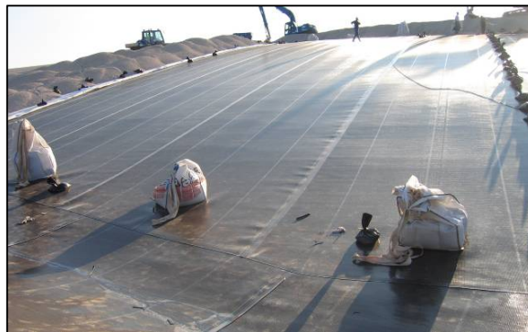
Figure 3: Lock bar installation, “Riegelbauweise”
