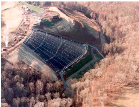
Figure 9. Site after installation of geomembrane
