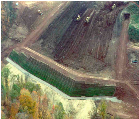
Figure 7. Placing impacted material behind MSE/CR buttress
