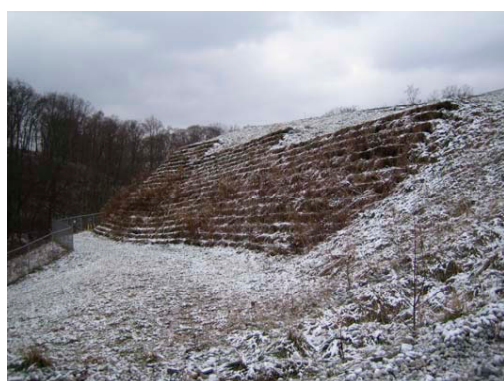
Figure 10. MSE/CR buttress in November 2005
