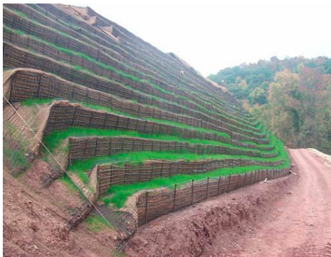
Figure 8. Front of MSE/CR buttress
