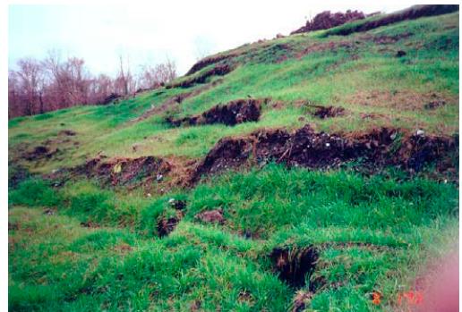
Figure 1. Site conditions in 1997 showing slide scarps at multiple locations
