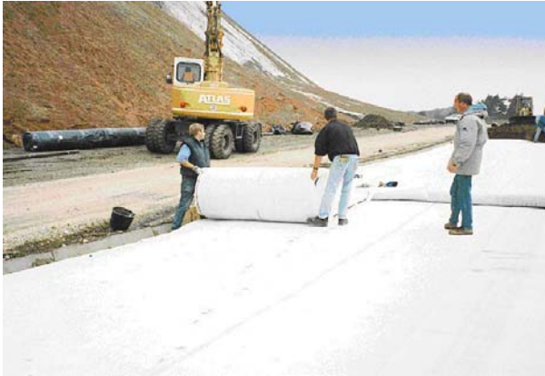
Figure 5. Shear strength transferring drainage geocomposite Figure 6. Drainage geocomposite on placement top of a GCL
