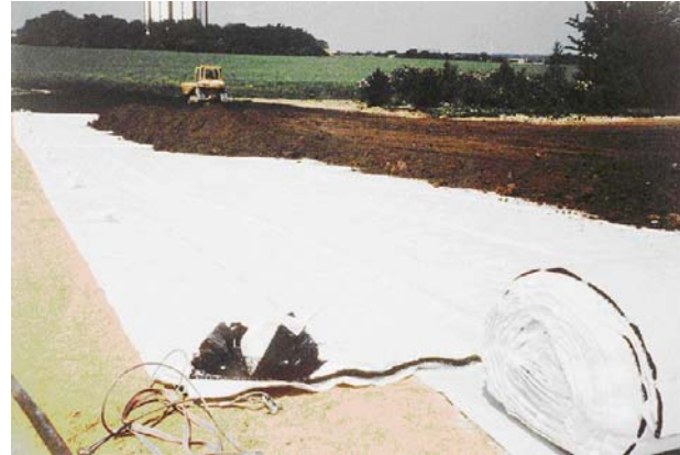
Figure 5. Shear strength transferring drainage geocomposite Figure 6. Drainage geocomposite on placement top of a GCL
