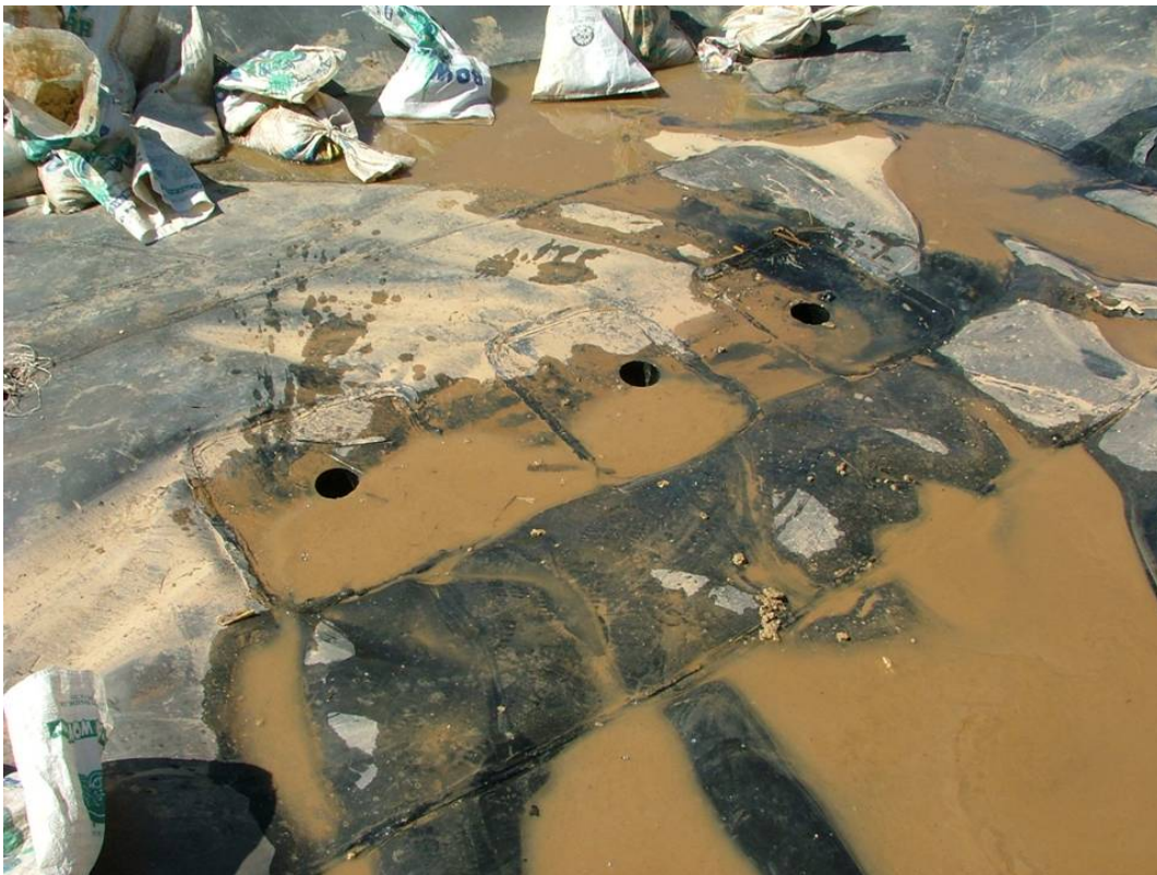
Figure 4. Leakage system outlets through the liner system
