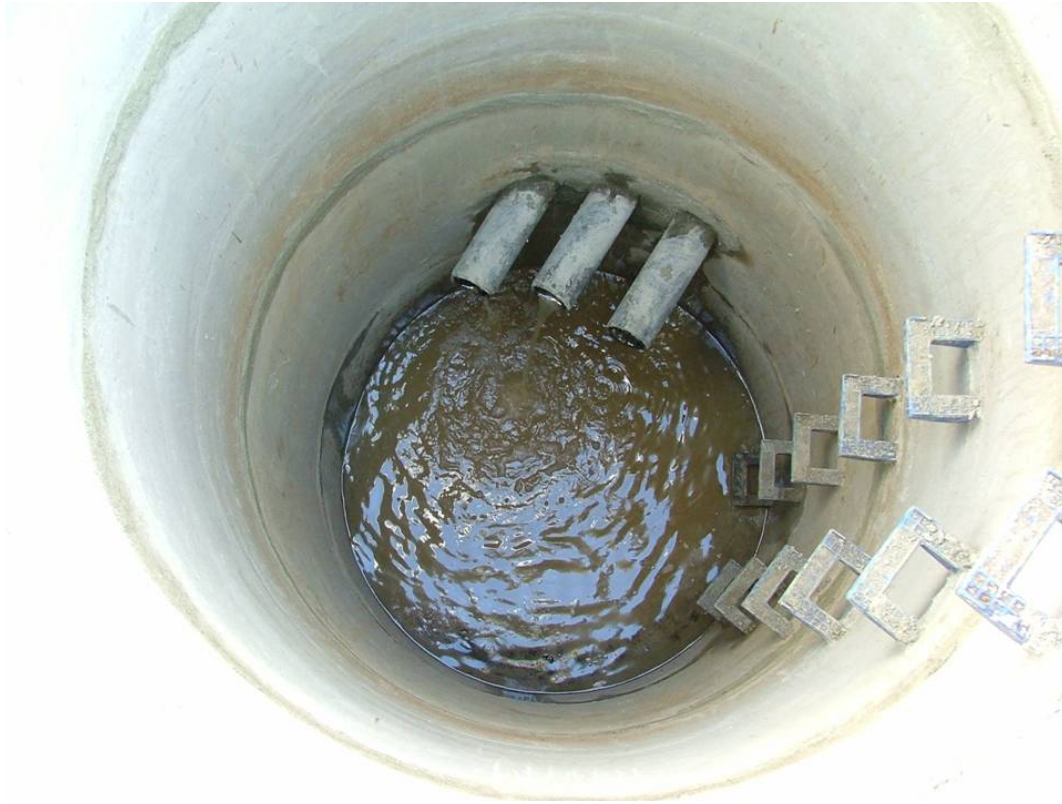
Figure 5. Leakage monitoring sump during construction
