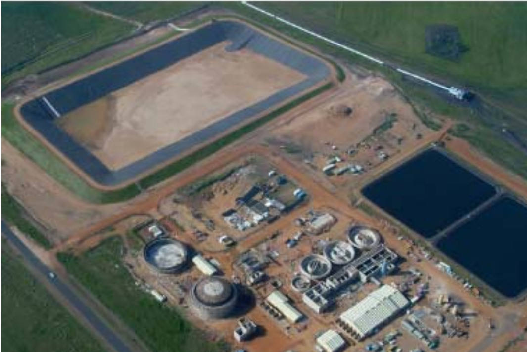
Figure 1. Aerial view of the brine evaporation pond and the water treatment plant
