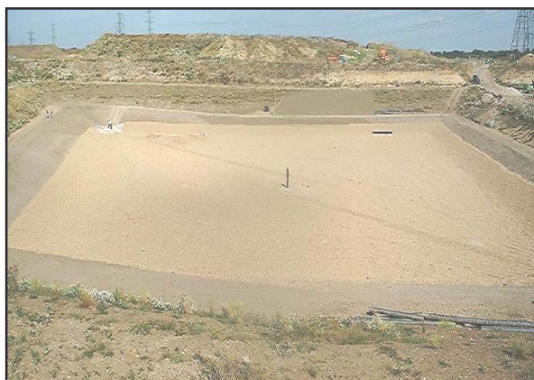
Figure 1. Cell 1B prepared for waste deposition
