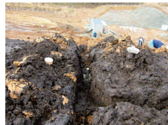
Figure 5. Covering soil sensor installation condition.
