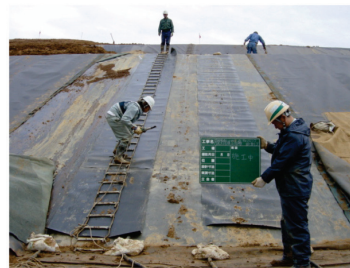
Figure 4. Sheet installation condition.
