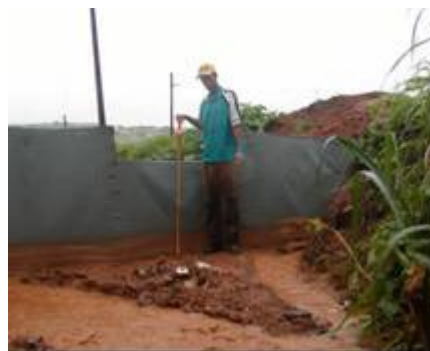
(b) Sediments retained upstream the fence
