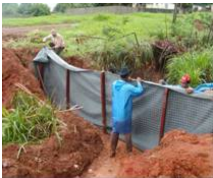
(a) Fence construction
